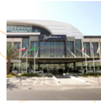
Radisson Blu Renovation
