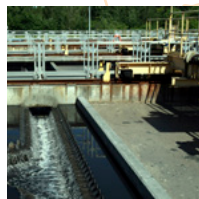
Seeb Wastewater Project
