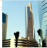
Al Hamra Firdous Mixed Use Complex
